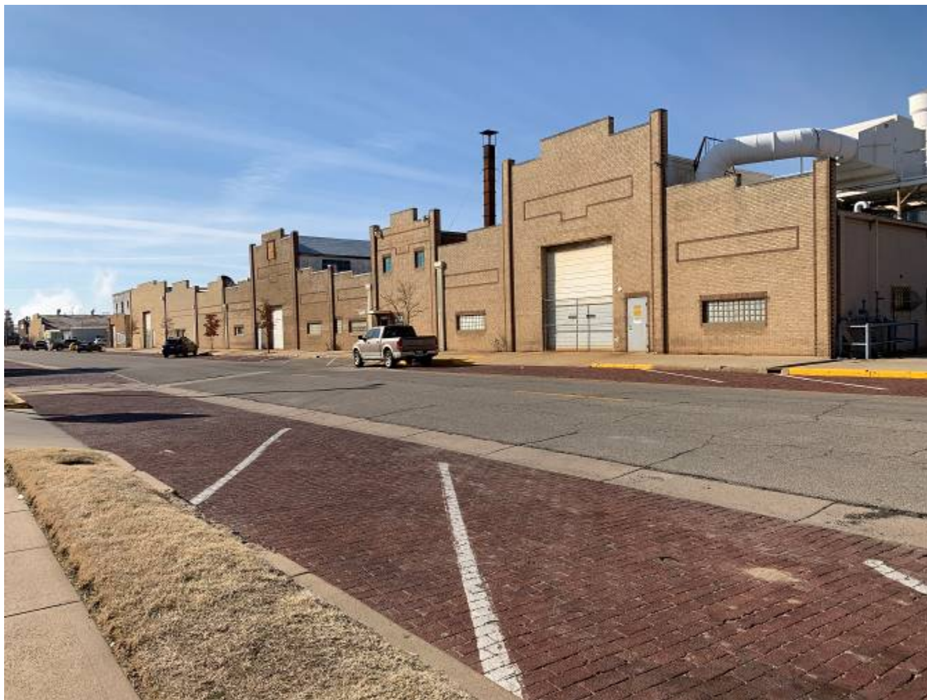
OK_Kay County_Nickles Machine Shop_0001
