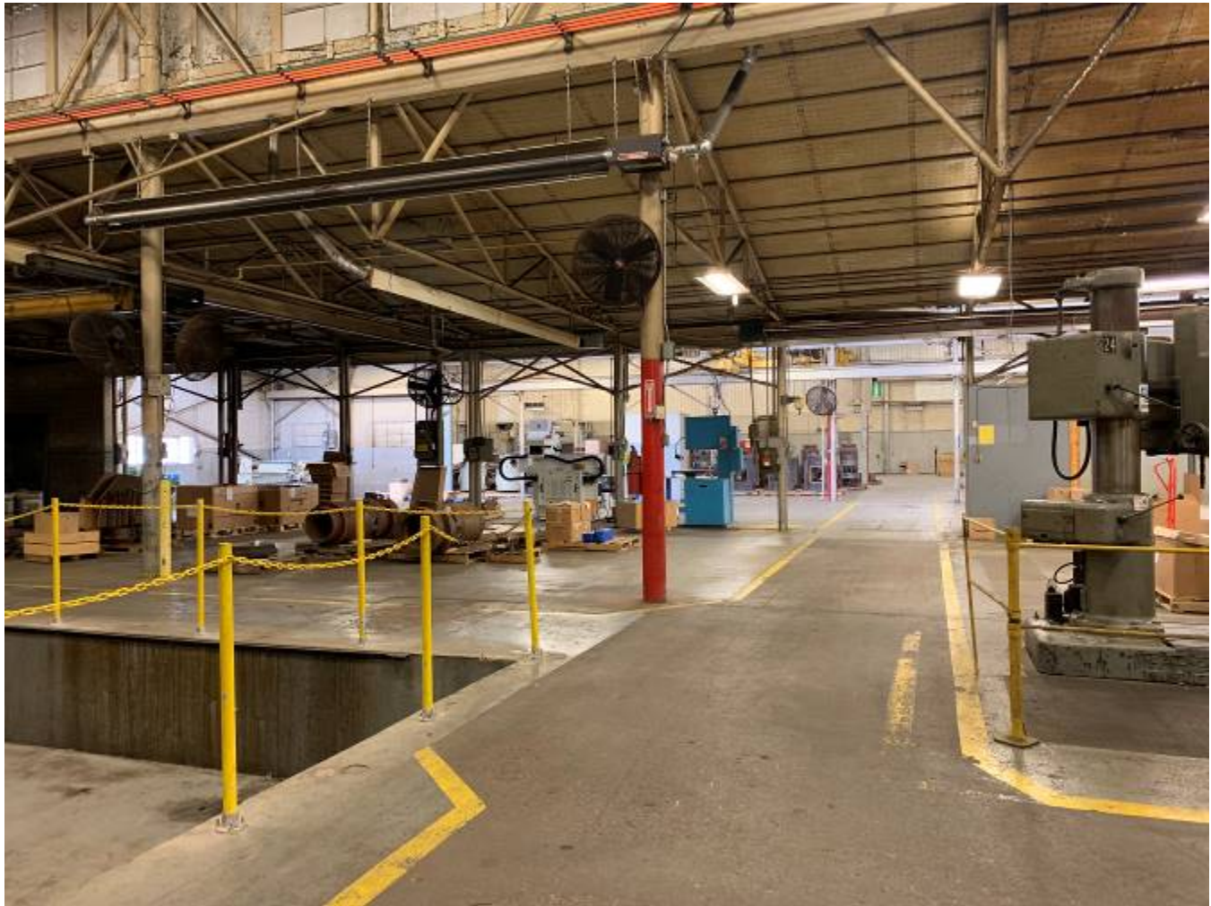
OK_Kay County_Nickles Machine Shop_0009
