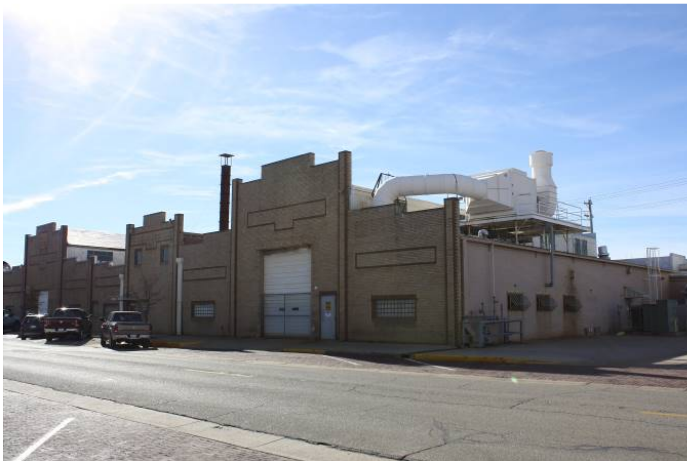
OK_Kay County_Nickles Machine Shop_0002
