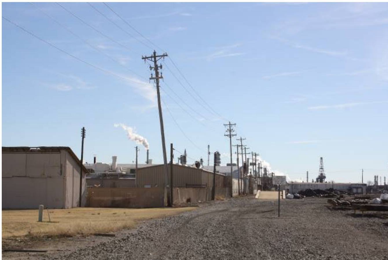
OK_Kay County_Nickles Machine Shop_0006
