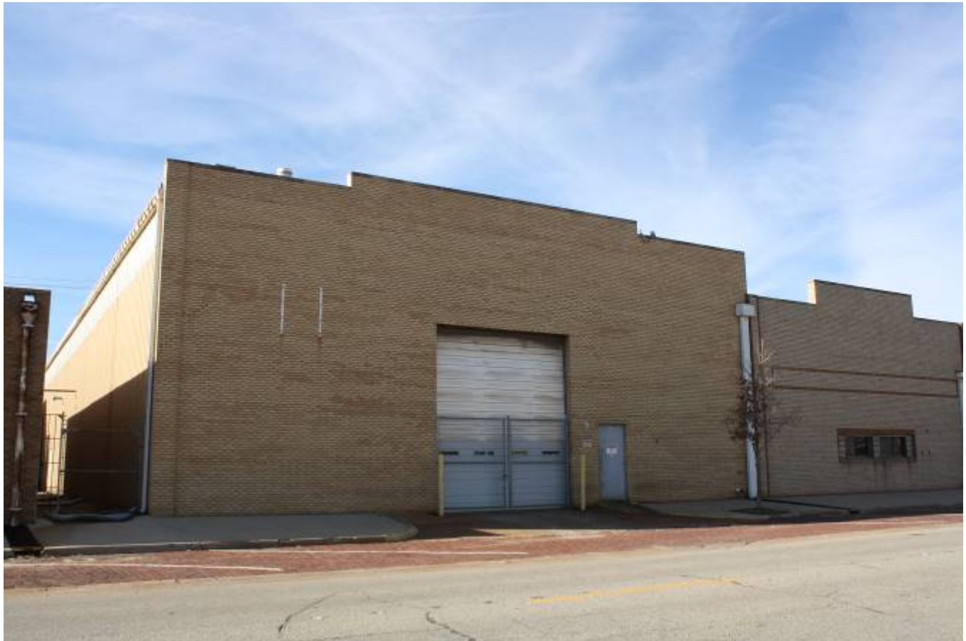
OK_Kay County_Nickles Machine Shop_0003
