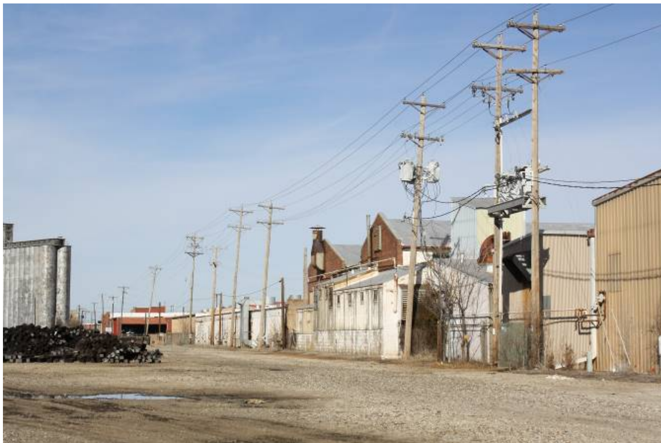
OK_Kay County_Nickles Machine Shop_0005
