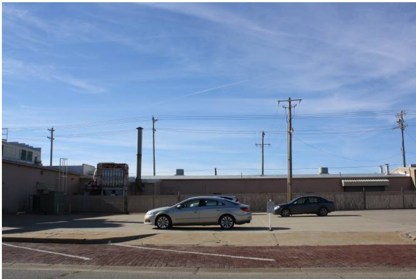
OK_Kay County_Nickles Machine Shop_0004
